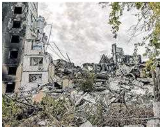
A view of apartment buildings damaged by a Russian military strike in Vuhledar, eastern Ukraine, last October.
