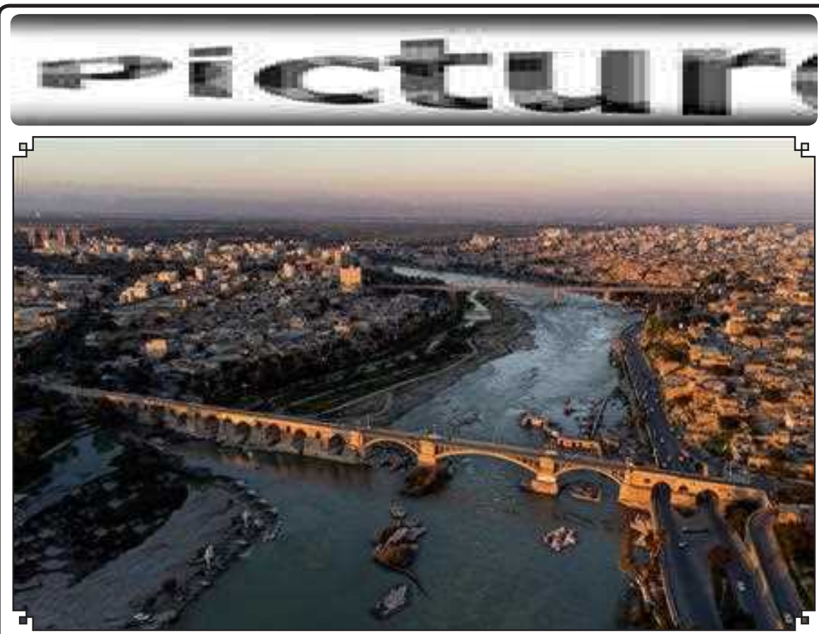
The Old Bridge of Dezful, connecting the western and eastern part of the city goes back to the Sassanid dynasty some 1700 years ago. However, its original foundation was built during the Elamite era.
