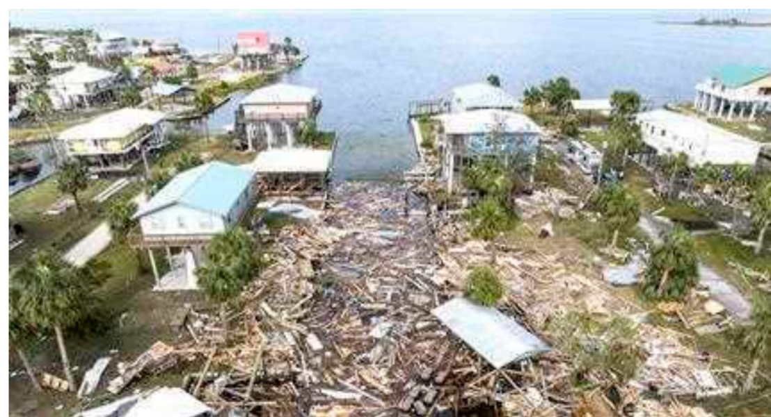
An aerial view of damaged houses are seen after Hurricane Helene made landfall in Horseshoe Beach, Florida
