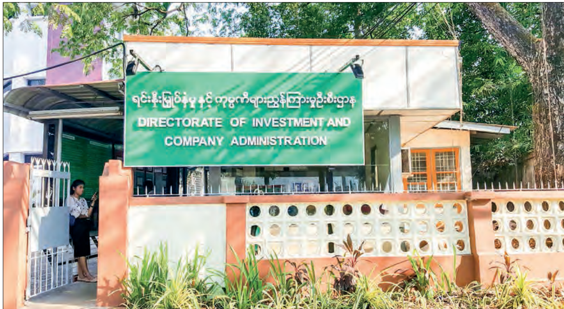
The facade of the Directorate of Investment and Company Administration (DICA) office.
