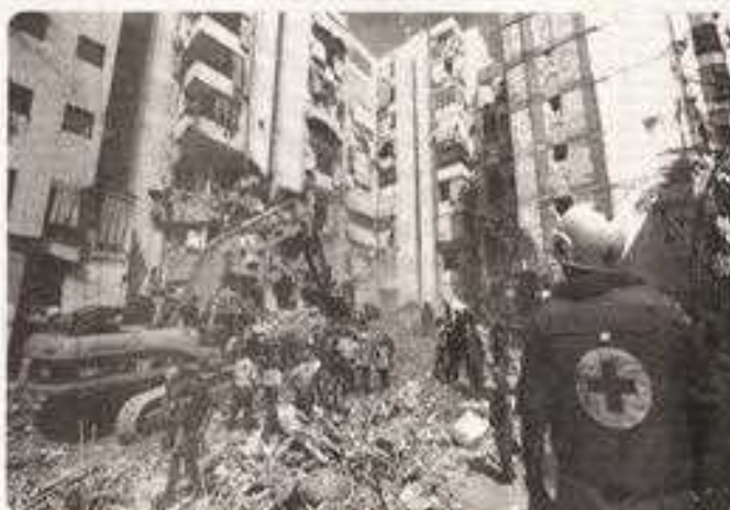
RESCUERS lifting through the rubble at the scene of an Israeli strike that targeted Beirut's southern suburbs.
