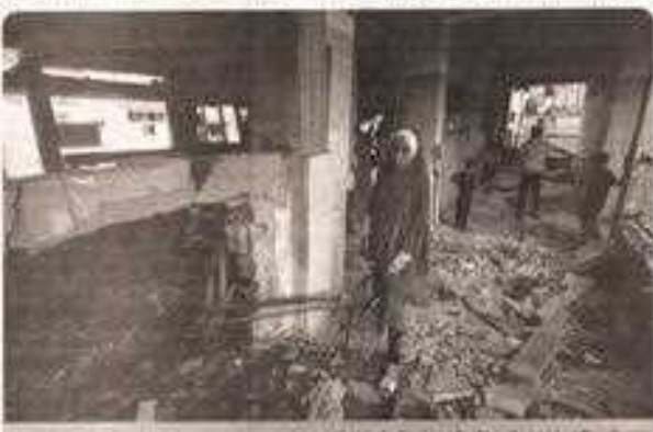
PALESTINIANS inspecting the damage to a school sheltering displaced people after it was hit by an Israeli strike at Gaza refugee camp in Gaza City, yesterday.
